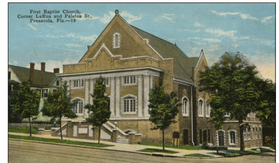
First Baptist Church, Pensacola
